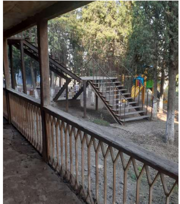
The metal staircase to the library. It was needed to add some segments of railing and rust protection.
