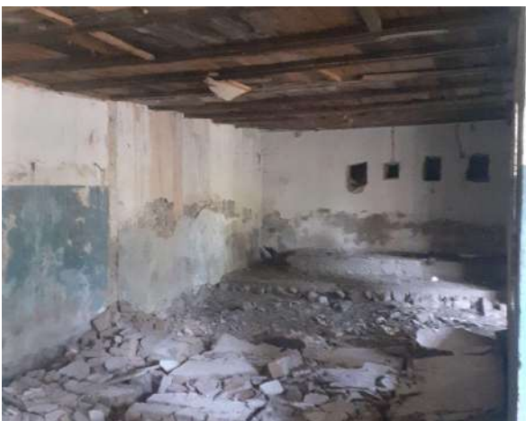
Existing room condition (1 st floor)
