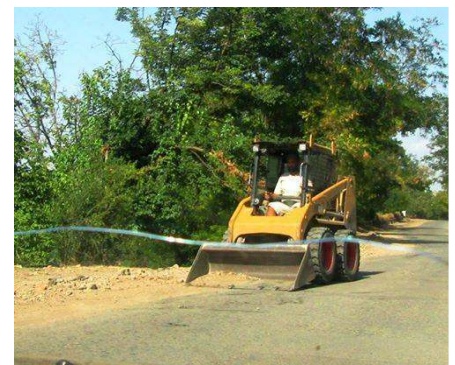
Local government of Marneuli organized work roads to improve the road to Tserakvi before One Caucasus 2014.
